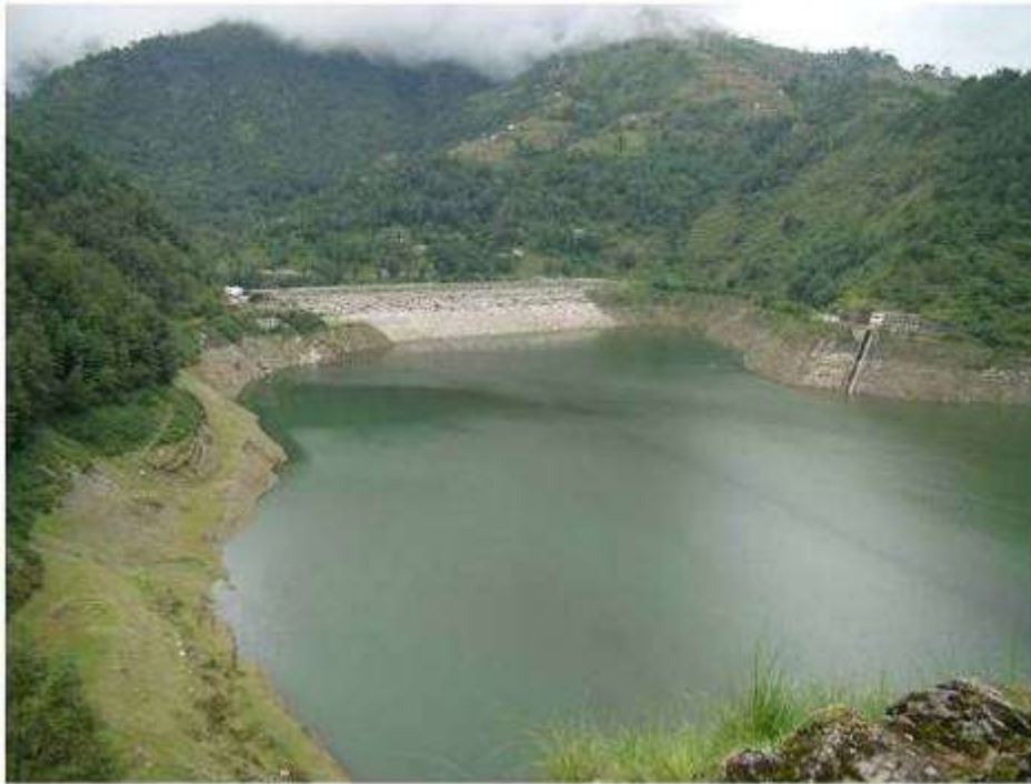
Kulekhani Reservoir: Level of water in the reservoir
